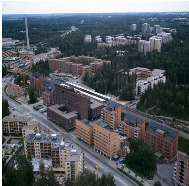
Figure1. Lassila under construction around the Pohjois-Haaga railway station at 1983. The Pohjois-Haaga tower blocks from the 50s can be seen in the back. (Scan-Foto, 1983.)
