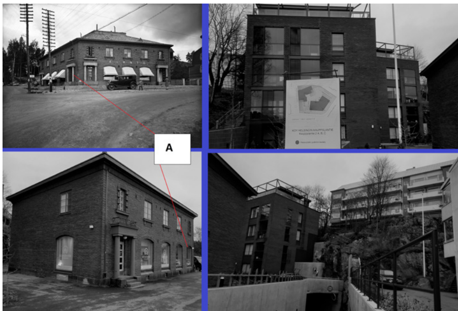
Figure 3. Elannon Liiketalo, Kauppalantie 2. Historical Photograph: Helsinki City Museum 1930 (Top Left). Modern Photographs: Rachel Jones Buildings to the west of Elanto building (Top Right). Elanto building photographed from south side (Bottom Left). Buildings behind Elanto building photographed from east side (Bottom Right).
