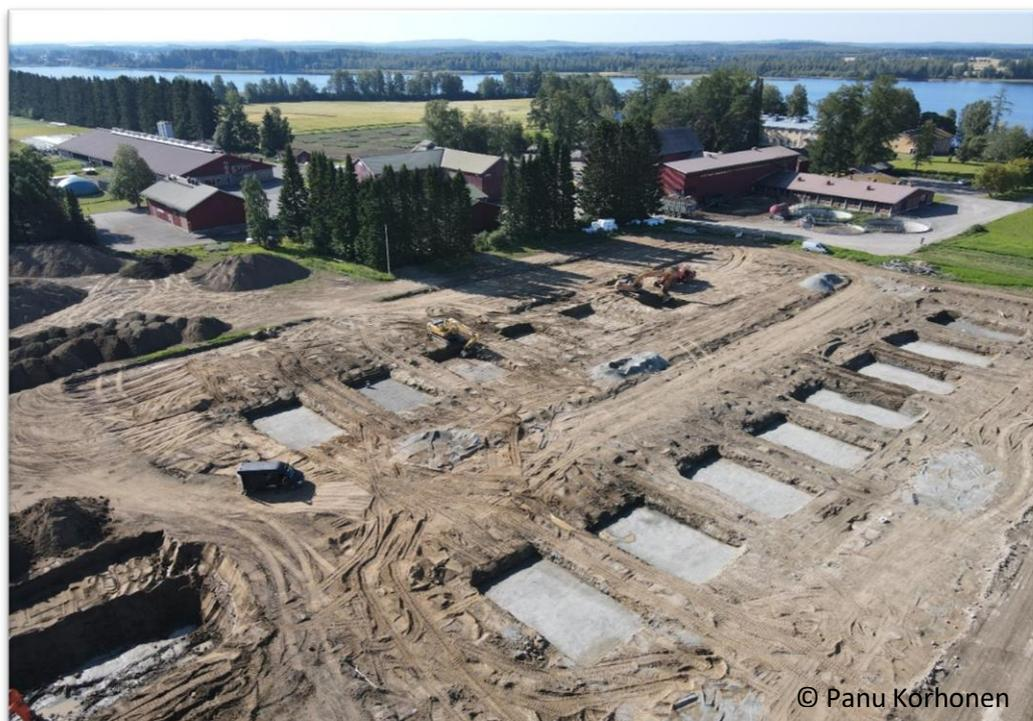
Figure 1. Building of the new surface runoff and lysimeter field at Luke Kuopio Maaninka station. It contains 16 individual study plots. The field will be in test use during summer 2021.
