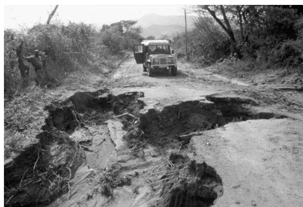
Figure 4. Rapidly extended gully has cut the road in Msau. (Photo: T. Sirviö)
