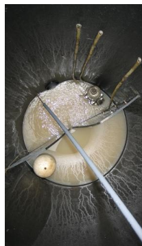
Sediment in the tile drain weir water
